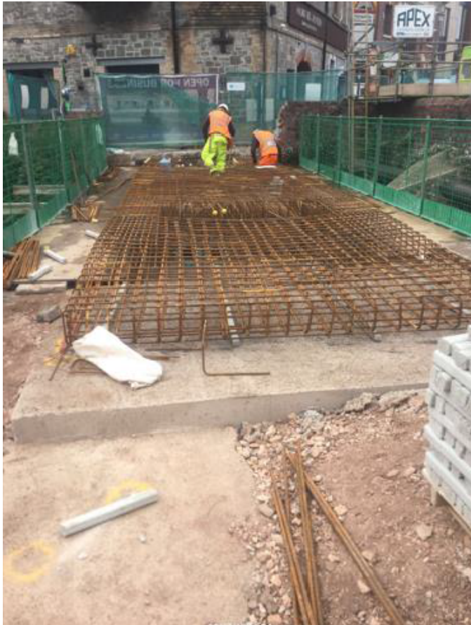
Deck being laid on structure across Cricklepit Leat at The Quay
