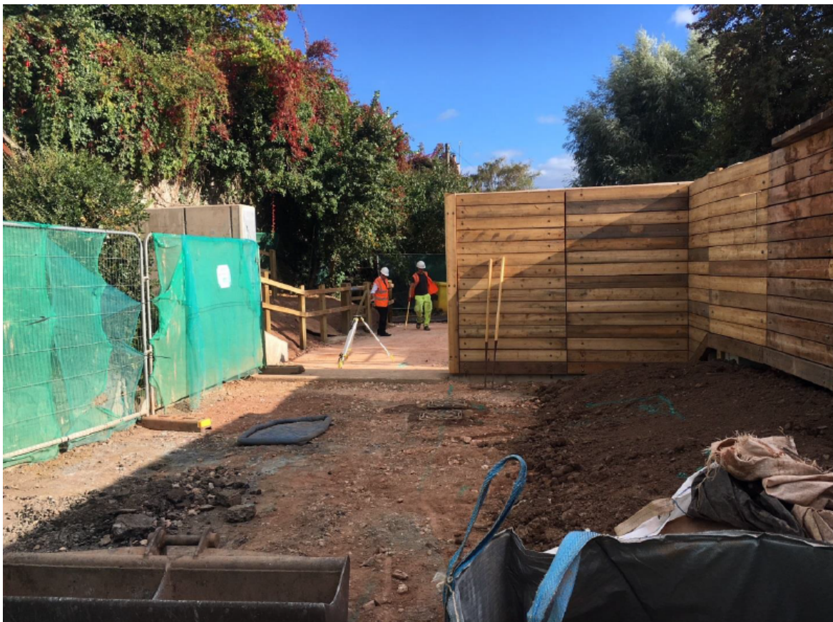
Mill Road flood gates under construction at Higher Wear (with new surfacing laid to the north)
